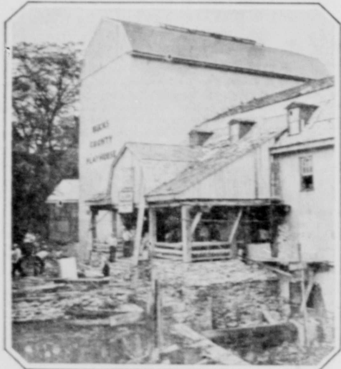
Once a mill, now a theatrical laboratory—the Bucks County Playhouse. Pipe at right diverts creek into showhouse cooling system.
