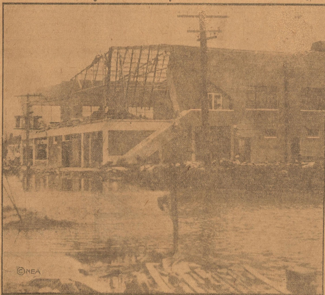
This theater building in Miami was literally ripped in half by the hurricane. The top and front were torn off and sent into the next block, leaving only a shell. Note how the street in front is flooded.
