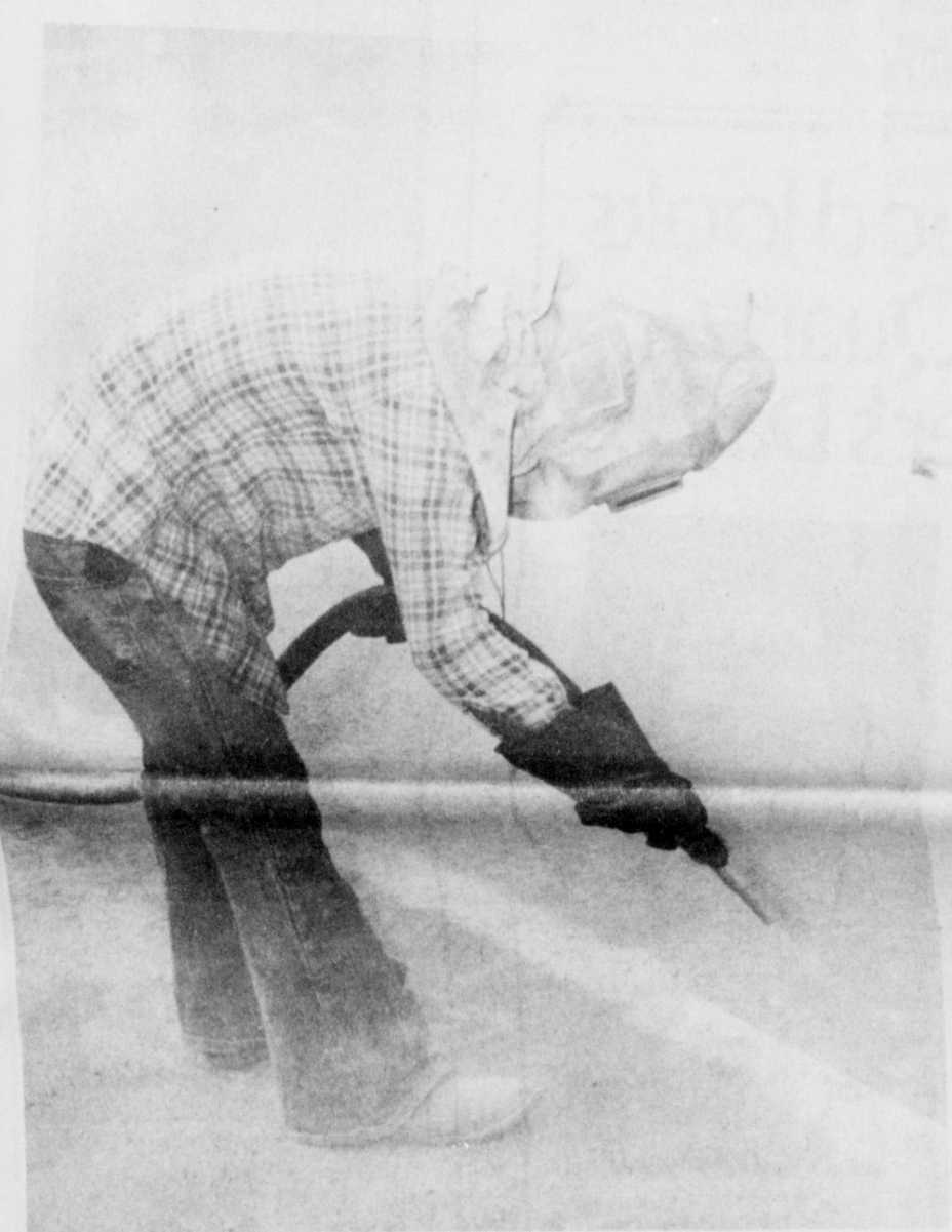
REMOVING PARKING LINES HOT, DIRTY WORK ... city employee at work on Cash Street.
