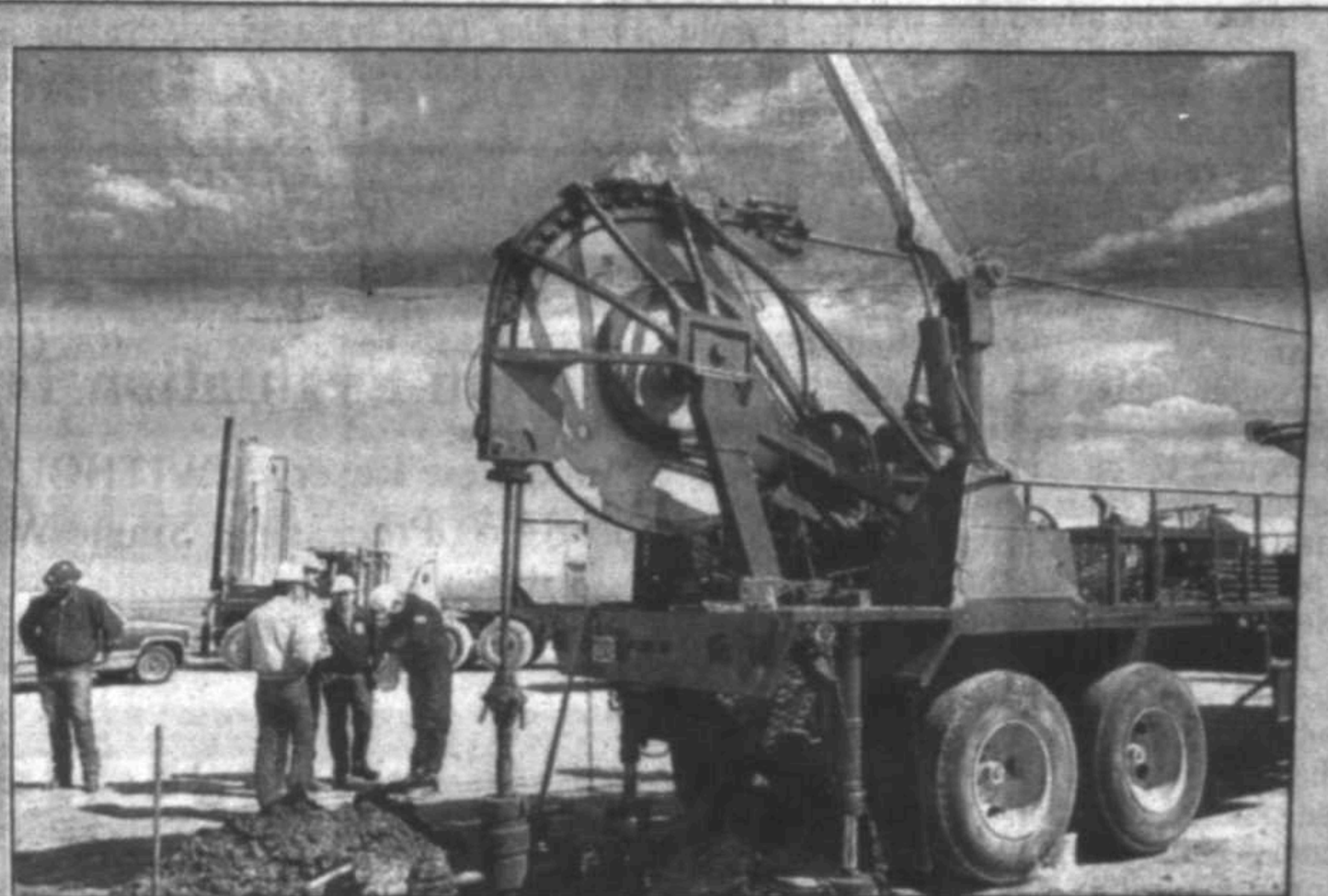
The CTU plugging rig seen above in an earlier test near Midland, could be the forerunner of a new coiled tubing application.
