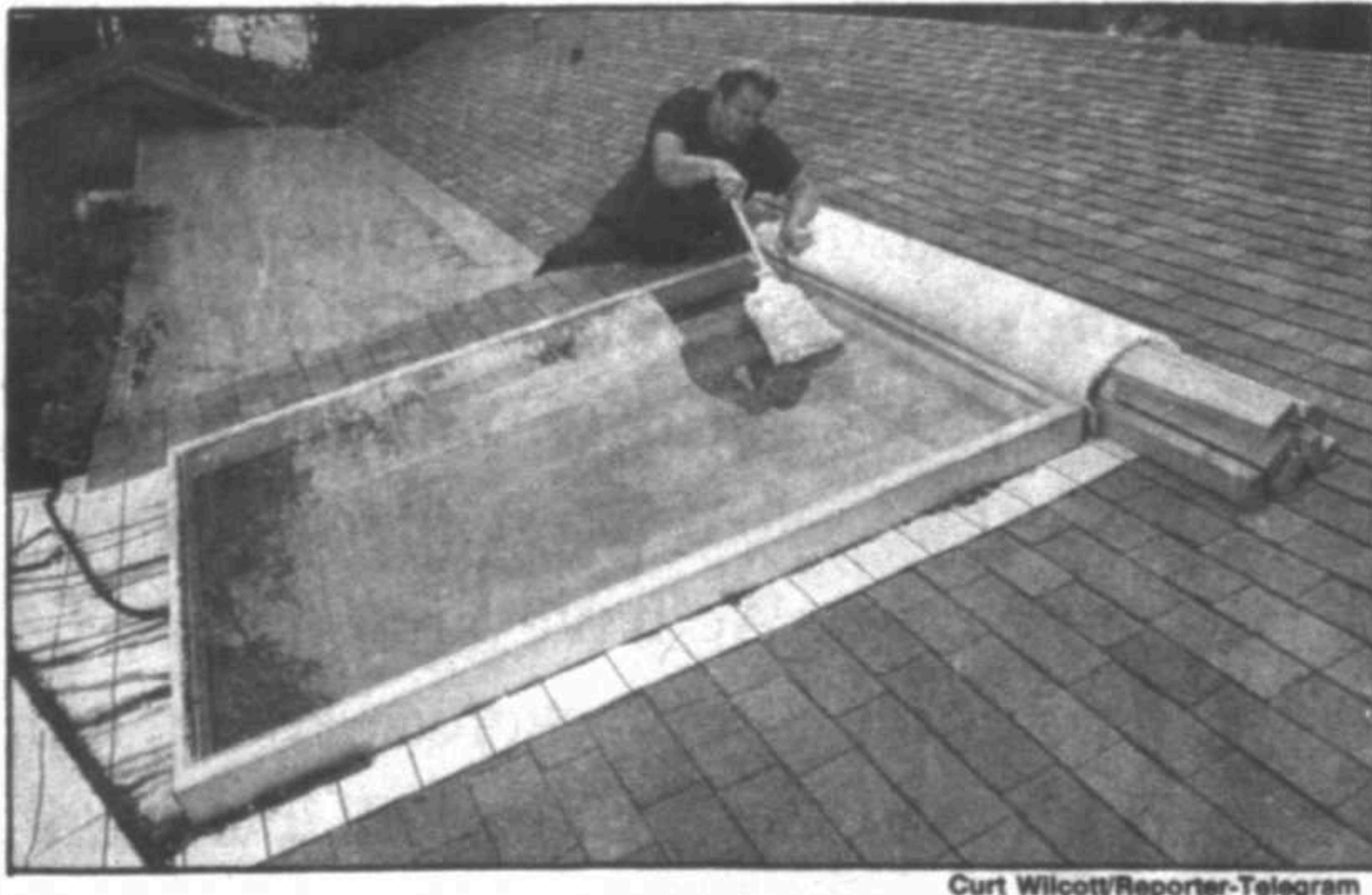
Steve Watlington cleans the glass of his roof-top solar still that produces about three gallons of distilled water a day.
