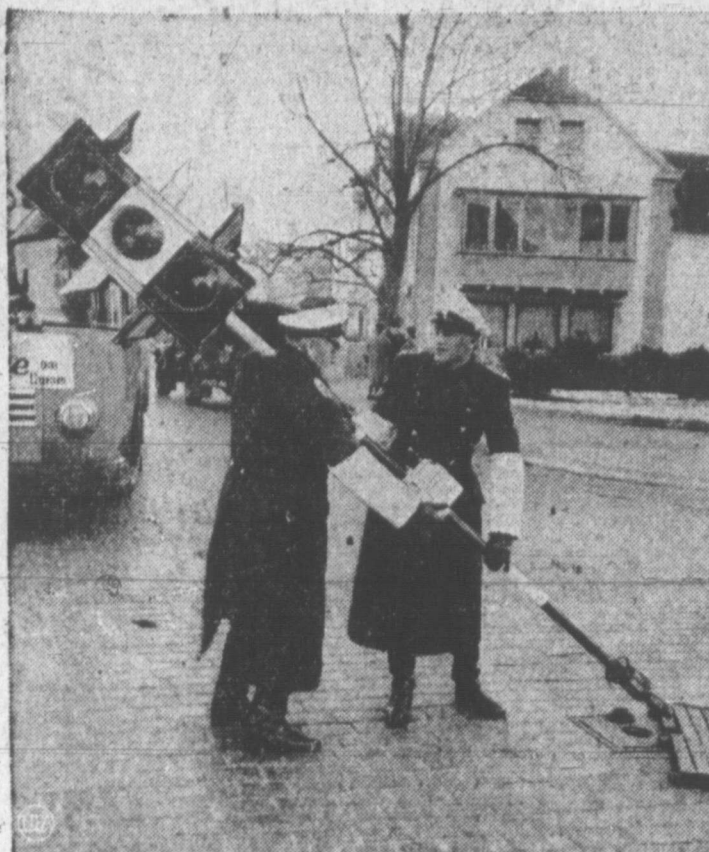
LIGHT WORK —Two policemen are erecting a plug-in traffic light at an intersection in Oldenburg, West Germany. Currently being tested in the city, the signal is held upright and supplied with power through the small opening in the street. Plugs at important intersections permit rapid installation of the portable lights when needed, as during rush hours.
