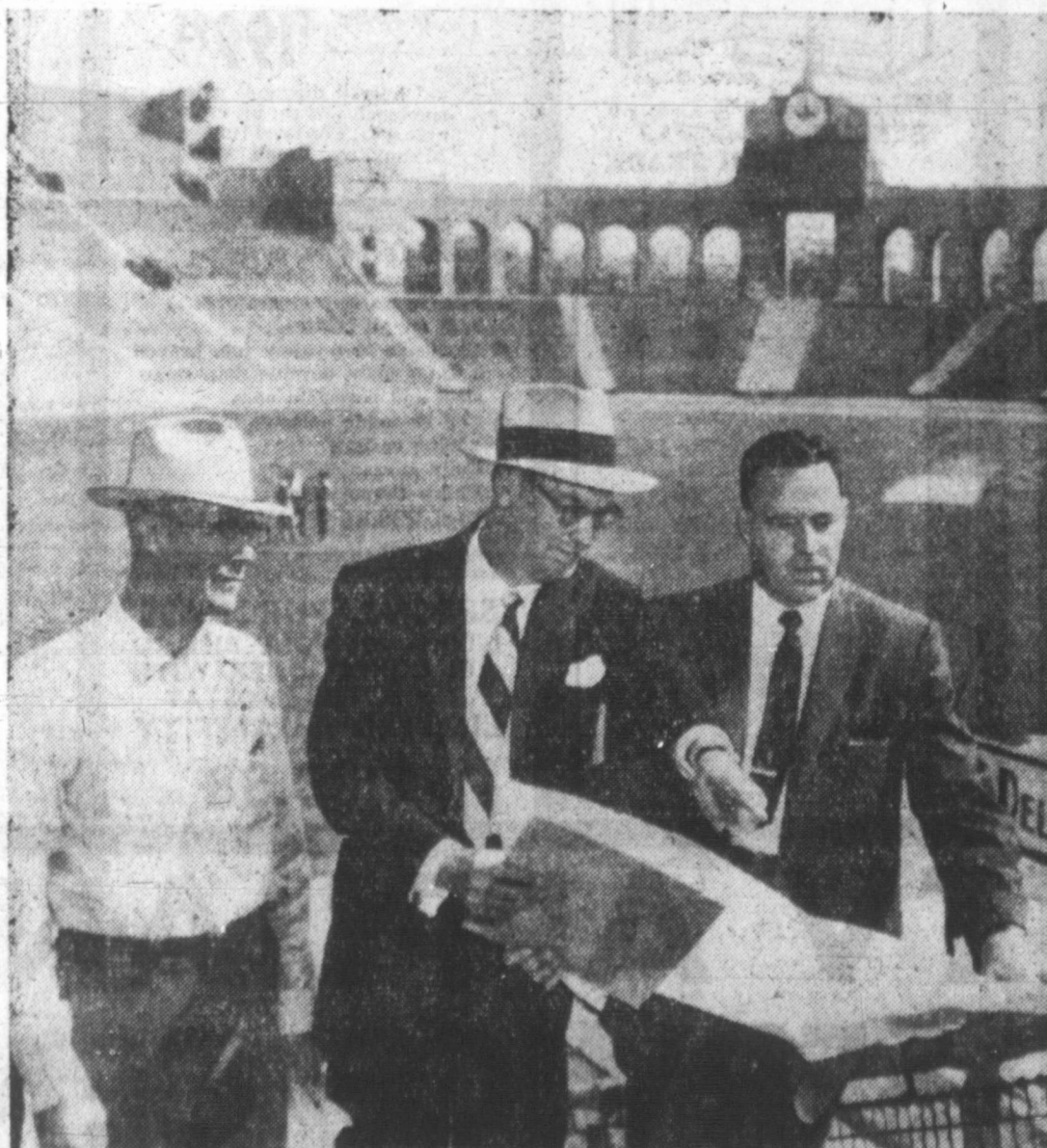
STARTING THE WORK —The construction work necessary to make the huge 103,000 seat Los Angeles Coliseum the home of the Dodgers is in full swing. Construction Superintendent Bert Broadhurst, left, and Ed Davies, right, confer with Del Webb, co-owner of the Yankees.
