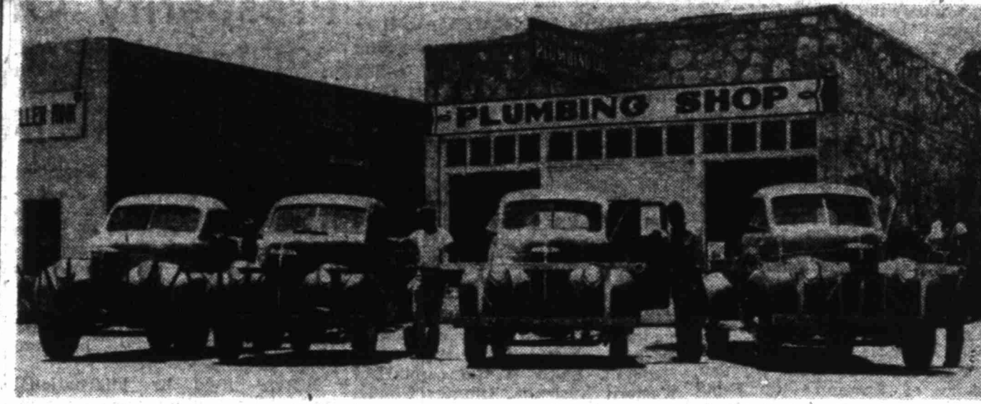
Heath and Templeton Plumbing Company's Midland store is being enlarged by the movement of the company's Odessa branch to Midland. This will give a sufficiently large staff of men and number of equipment units to serve the entire Permian Basin from Midland. The men and trucks pictured here are only a few of those which will operate from Midland when the merger of the stores is completed. Oil-field, commercial and residential plumbing contracts anywhere in this part of the state will be a specialty of the firm. Left to right in this view are Johnny Cryer, Jay Francis, Maurice Conrad and Jim Grady.
