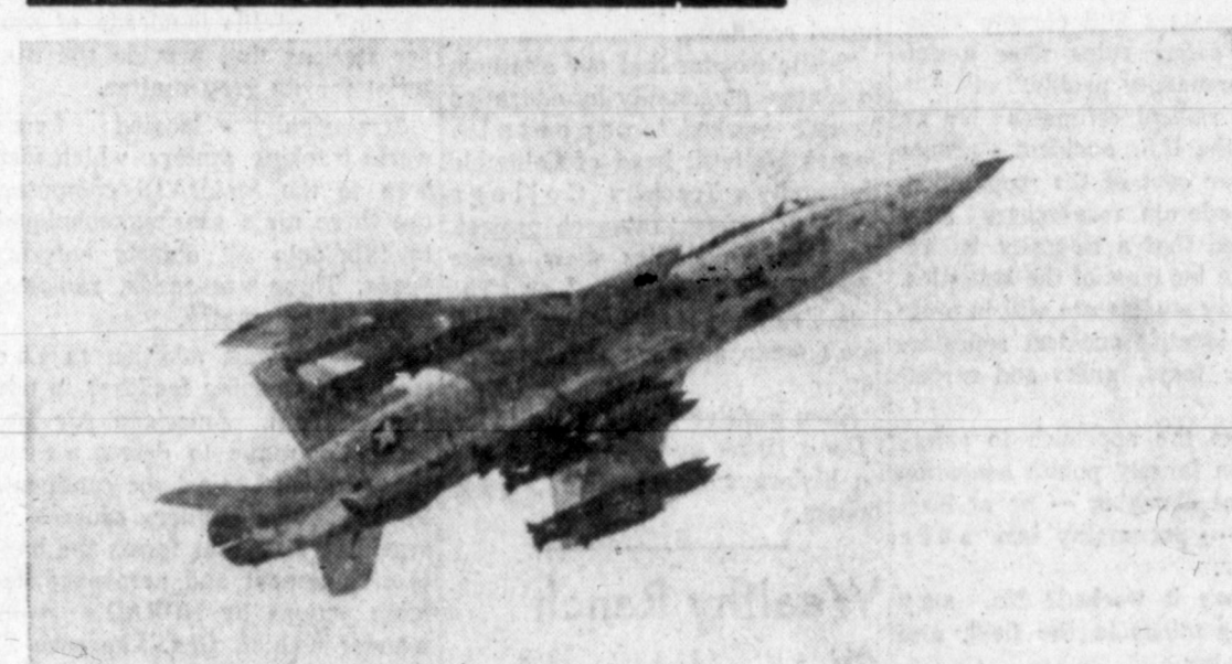
BOMBER BAGGAGE —This Republic F-105 fighter-bomber is carrying seven tons of non-nuclear bombs in a demonstration of limited-war mission. The 26,565-pound bombs, mounted on wing and belly racks, is the largest load ever flown by a single-engine fighter.
