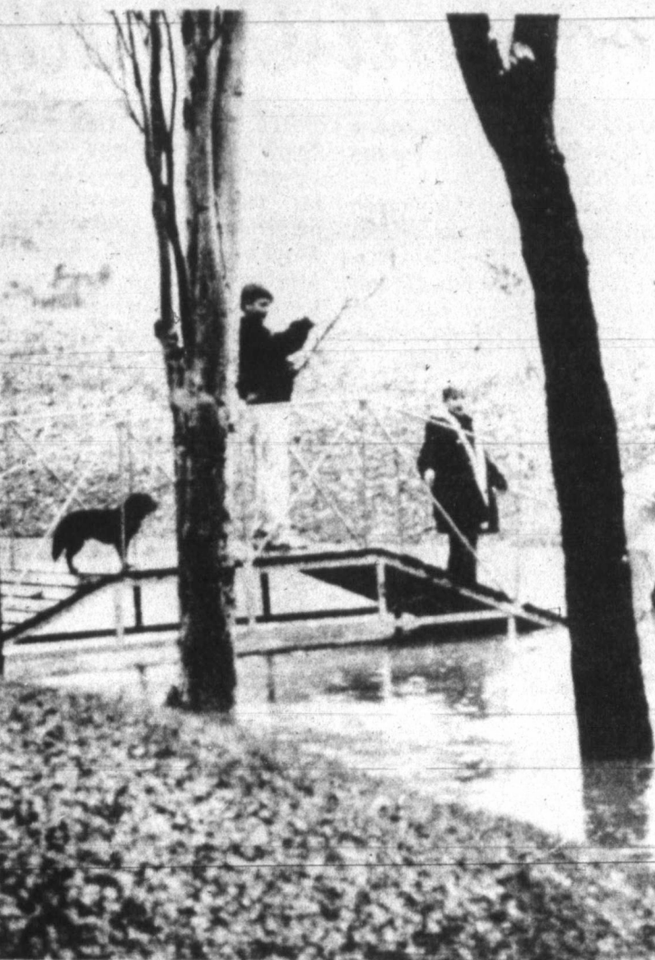
BRIDGE DOWN—This bridge across Red Deer Creek in Central park was washed away from the bank by yesterday's high water. The photo
