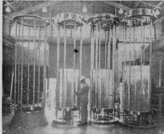
PLANNED FOR POWER —Technician adjusts a core structure at the National Reactor testing station near Idaho Falls, Idaho. Plant is to test the feasibility of making super-heated steam by utilizing uranium fuel to drive power-producing turbines.
