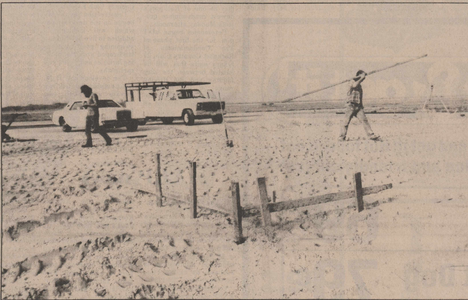
WORKERS PREPARE TO POUR a new slab behind a slab poured too close to a
