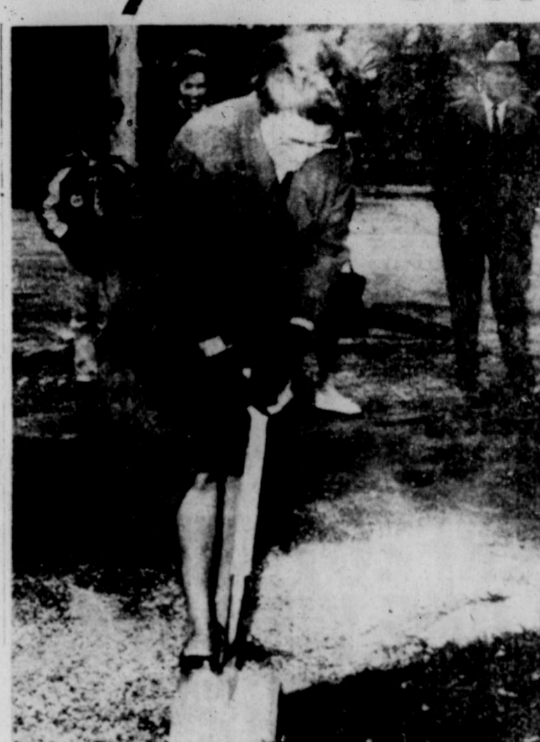
The Beginning OF CONSTRUCTION on the new Mitchell County Library was initiated by Mrs. George Witten, county library board president, as she turns over the first soil at the building site.
