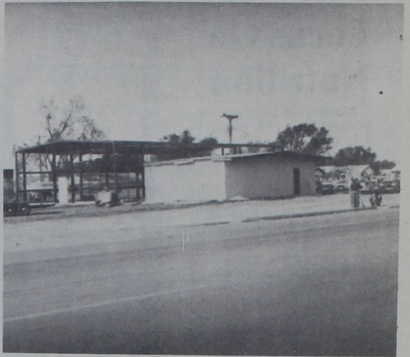
CONSTRUCTION UNDERWAY... Work is underway on east Highway 60 for a truck wash facility. Hack Corbell is installing a truck wash. Details on completion, etc., will be forthcoming.
