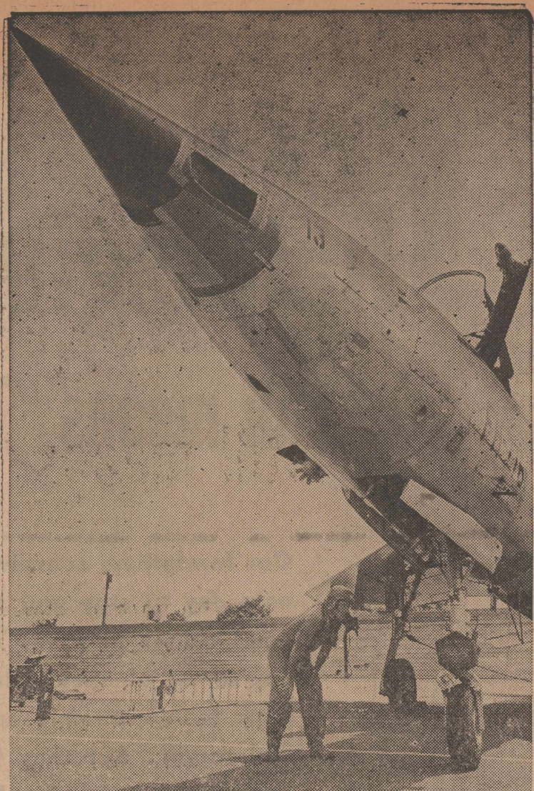
NOSING SKYWARD —As sleek as a sharpened pencil point, the nose of a Republic F-105 Thunderchief towers over test pilot Carl Ardrey at Fannin, N.Y. The pilot is studying a new steering device built into the nose wheel of the Air Force supersonic fighter-bomber.
