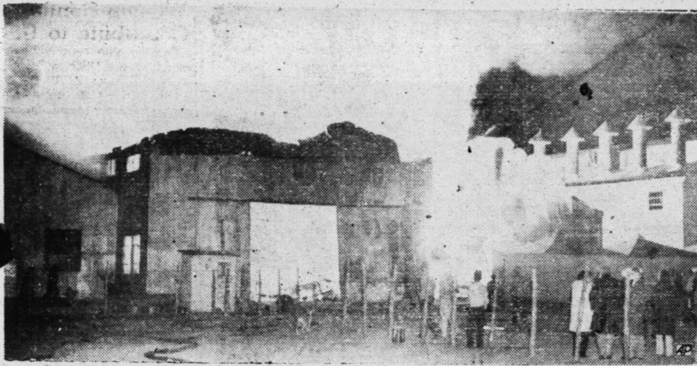
FIRE SWEEPS DALLAS DEFENSE PLANT — The Austin Bridge Company plant at Dallas, which manufactures incendiary bomb cases was heavily damaged by a fire which destroyed thousands of dollars worth of vital war materials. This photo was taken while the fire was at an early stage. The glare was so bright it could be seen for 80 miles.
