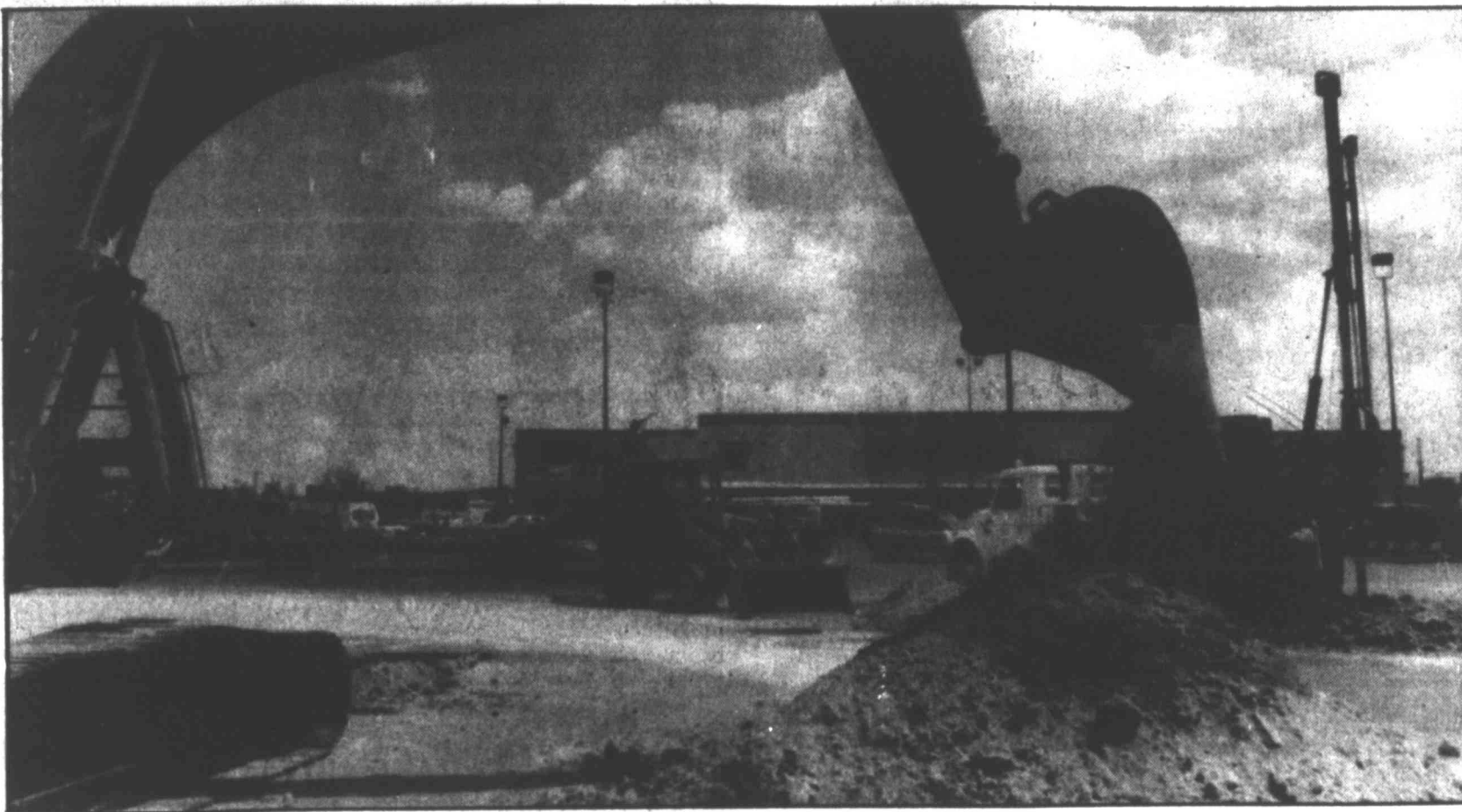
Heavy equipment tear into the asphalt and dirt underneath on the north side of the HEB parking lot Tuesday afternoon. Work began at the site Tuesday on the construction of a new gas station operated by HEB. Similar stations at HEB stores in Abilene and San Angelo have seen gas prices plummeting in those areas.
