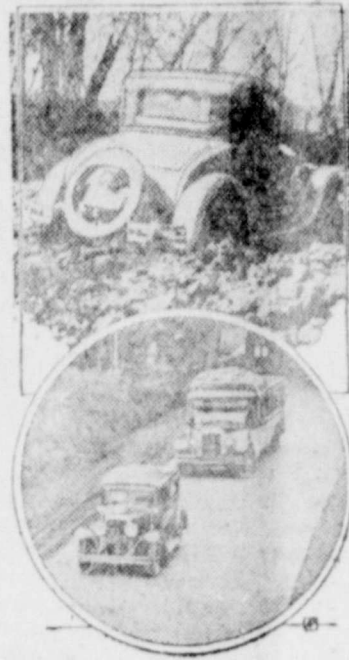
Highway rousecleaning in Iowa is nearing completion. Typical Iowa mud road (top) is compared with one of the state's new hard surfaced highways.
