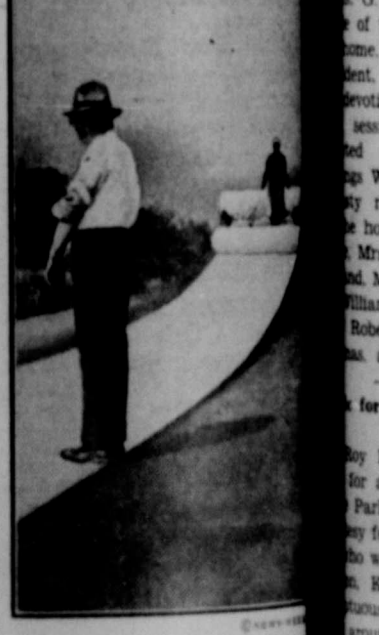
SOUTH'S COTTON ROADS As an outlet for surplus cotton, southern states have laid 500 miles of cotton-reinforced highways. Cotton base prevents cracks and erosion.
