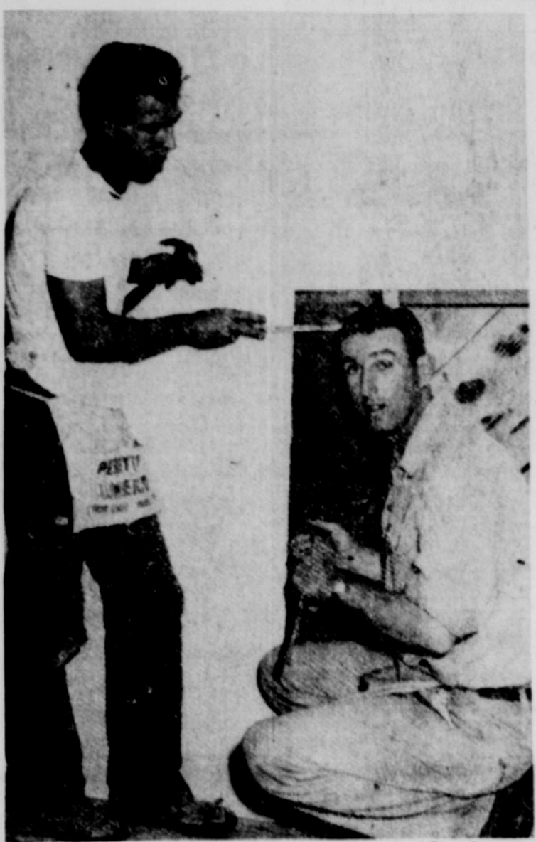
MEN AT WORK —What do school teachers do during their summer vacation? These two have been putting in about 15 hours a day on carpenter work, building a couple of houses. They are Earnest Kendrick, left, assistant coach, and Kenneth Gibson, right, high school principal. They each have a house under construction in the Stark addition and hope to have them completed by fall. Neither teacher is a carpenter, but are furnishing the labor under the technical direction of contractor A. J. Zedja.
