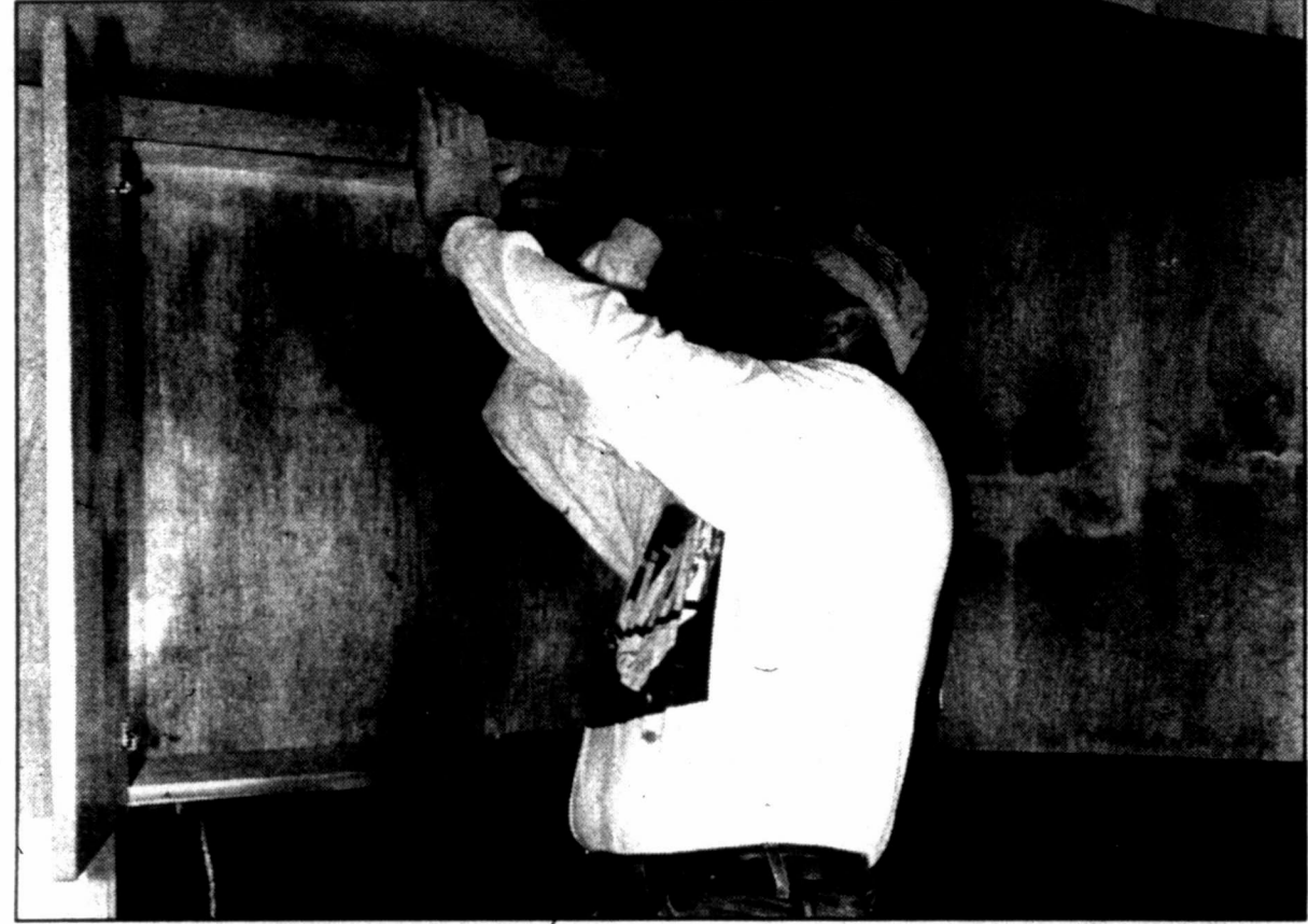
CABINET PAINTING is part of the finish work remaining in fieldhouse addition construction at Wolf Stadium. Curtis Mann of Snyder, an employee of paint contractor Robert Greene, applies elbow grease to sand down the cabinets in preparation for the painting.
