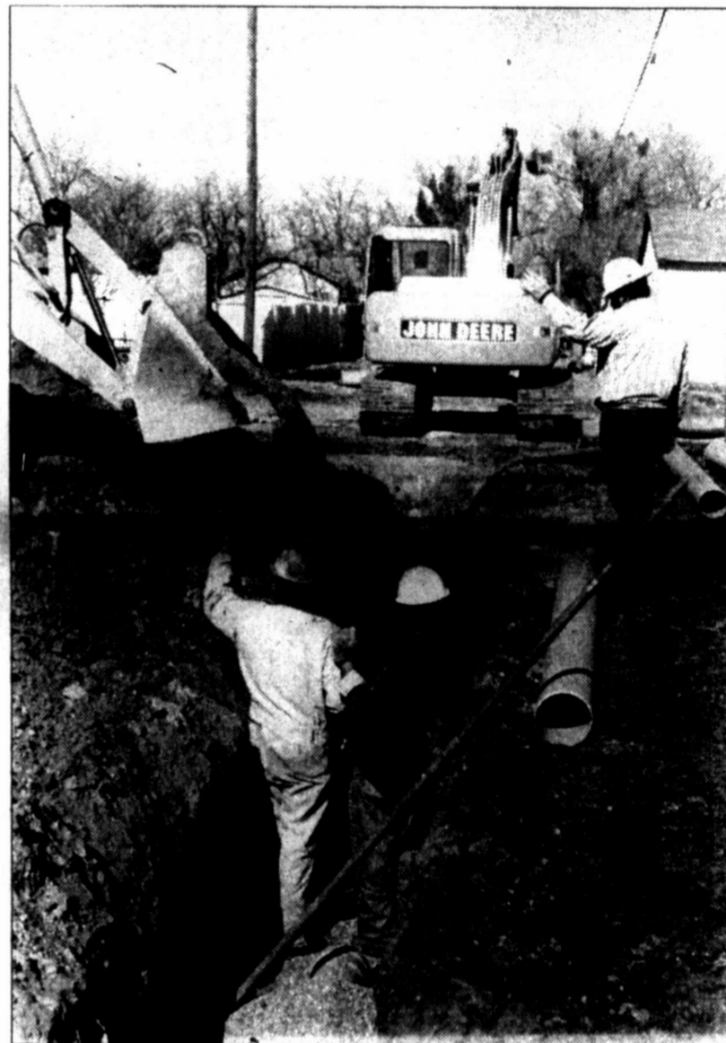
ROBERTS CONSTRUCTION CO. workmen from San Angelo were busy laying a new sewer line Friday at Seventh Street between Walnut and Oak Streets. They will lay it to 17th Street and then east toward Mitchell County Hospital. They are Greg Macias, top right, Manuel Meza, in the plaid shirt, and Flaco Cruz.
