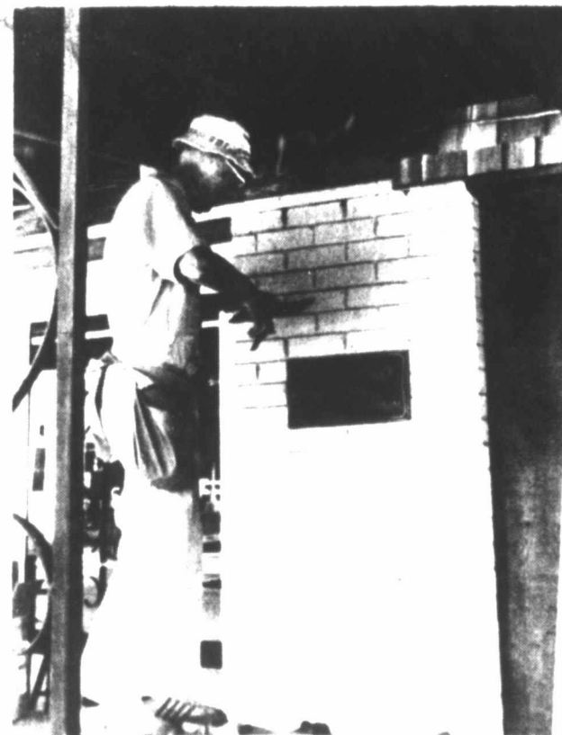
JOHN TOM MERRITT puts the final touches on the front of the Colorado City Museum as he completes renovation work on the building, located on the corner of Third and Oak Streets.
