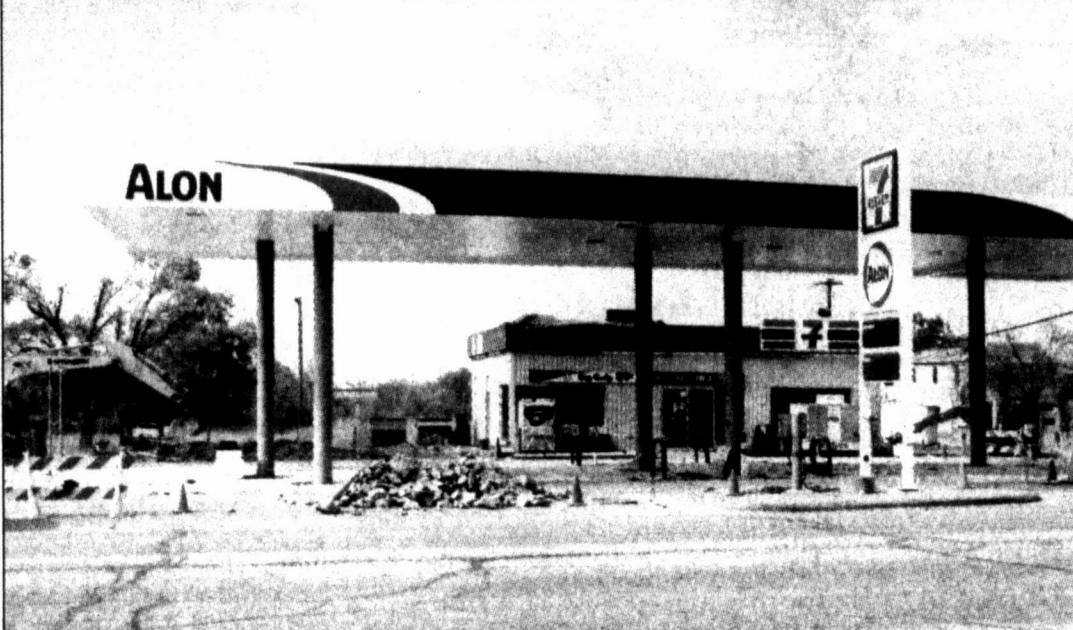
BRING ON THE FUTURE — Alon USA has undertaken a complete renovation and expansion of the 7-Eleven convenience store on 2nd Street in downtown Colorado City. The store will be closed from July 19th until August 2nd to allow for upgrades inside.
