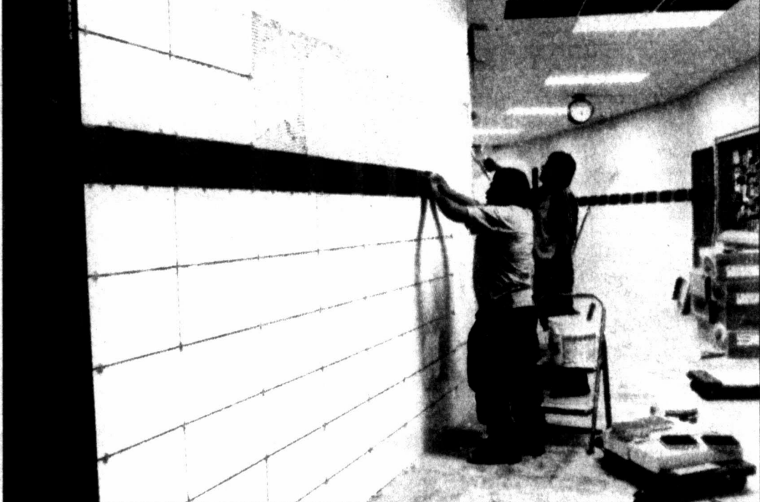
A NEW LOOK — Workers from All Commercial Floors in Arlington install new ceramic tile along the walls of Colorado High School. Charlie Price of Compass Builders says that work is on schedule and should be finished before the first day of school on August 25th.
