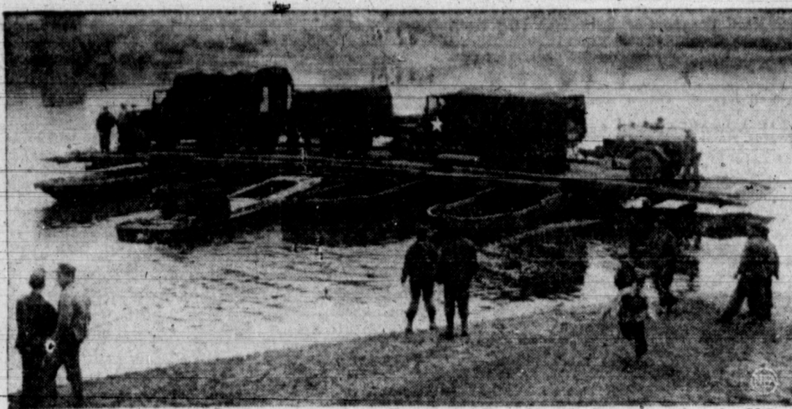
ACROSS THE RIVER —Across the Mosel River near Bern-Kastel, Germany, goes the U.S. Army's heavy equipment assault boat. It's powered by the inboard-engined motor boat in the center. This is standard procedure for moving vehicles across a river. This was part of Eighth Infantry Division operations.
