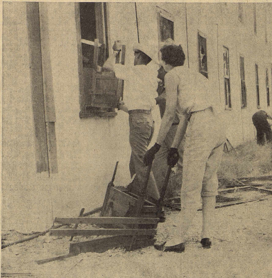
HEAVE IT UP was heard Wednesday morning as local workers met at the old hotel and pitched furniture and fixtures back into the building.
