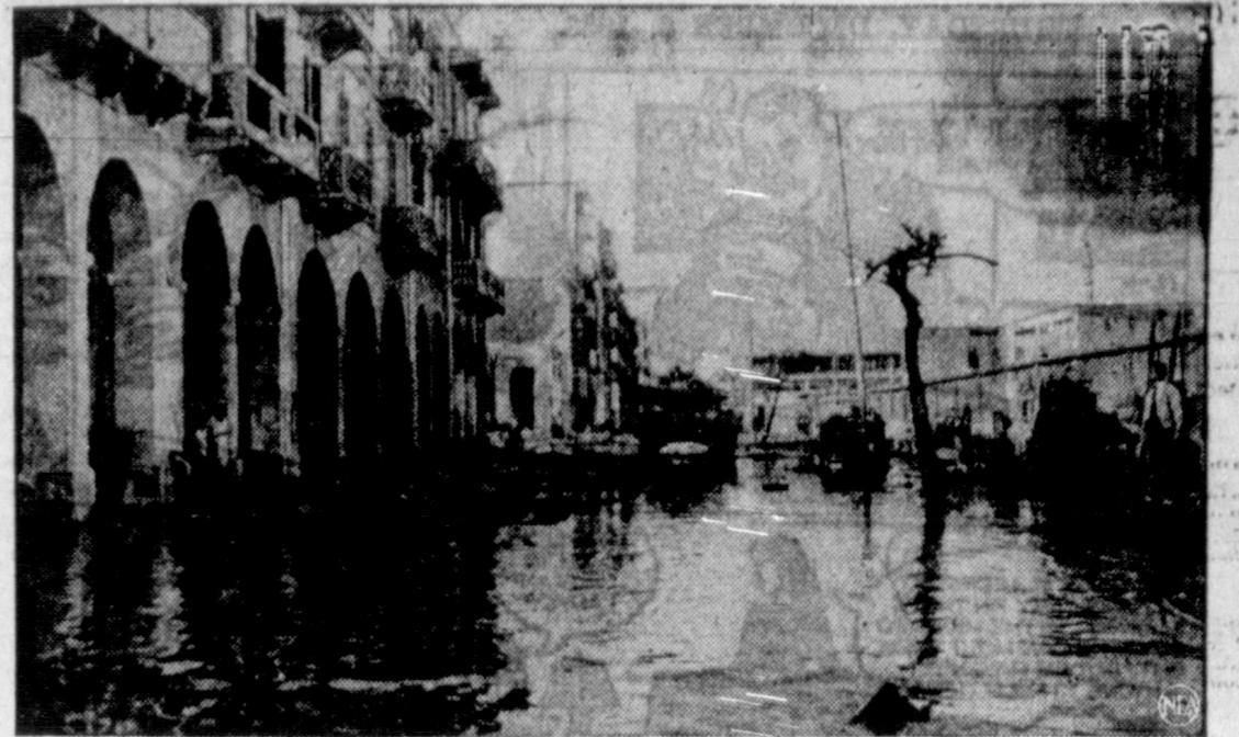
VENETIAN SCENE —Looking like a vista along the Grand Canal in Venice is this picture of a flooded street in Port Said, Egypt. Civilians try to salvage their belongings from wrecked buildings while a British tank stands guard.
