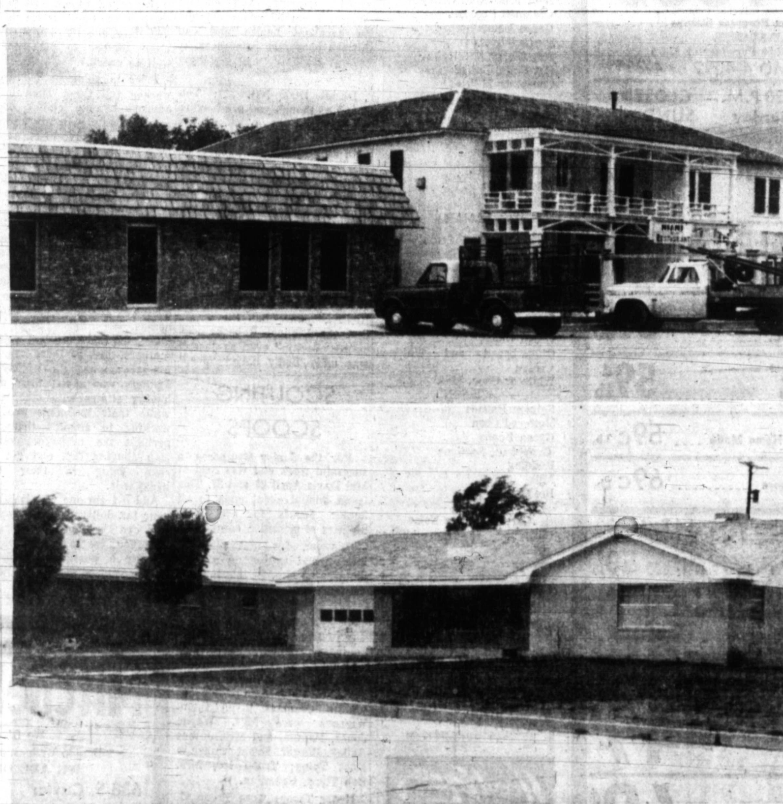
COMPLETELY REBUILT — Although struck hard by a tornado May 6, 1968, all buildings and homes in Miami have rebuilt. In the top picture the gas company on the left was demolished by the twister and part of
