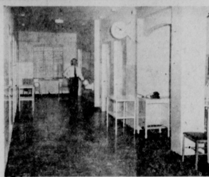
INTERIOR OF HOSPITAL—J. D. Everett, business manager of the Sanford Hospital and Clinic, is shown above in the second floor hall. To the left is the nurses call station and the diet kitchen is on the right.
