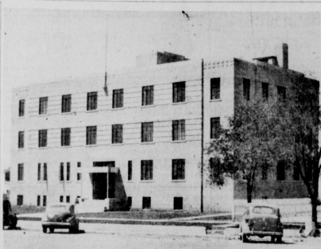
NEW HOSPITAL AND CLINIC—Exterior view of the Sanford Hospital and Clinic which will be opened to the public on Saturday, May 17. The architectural design was done by C. L. Monnot of Oklahoma City and construction of the building was done by the Manhattan Construction Company of Muskogee, Okla. The hospital is located across the street from the Ochiltree county courthouse, facing east.
