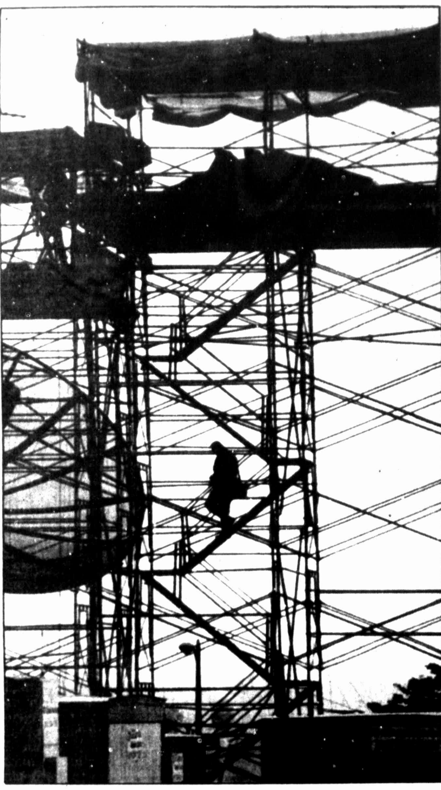
Los Angeles Times photographer Axel Koester makes his way down from a news scaffold across the street from the Criminal Courts building Sunday. News media from throughout the world have set-up a field camp across the street from the courthouse.
