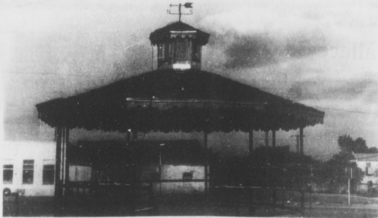
THE GAZEBO, being built at Dell Barber's Kiwanis Park is taking on a real look of a gazebo. Work has stepped up, but was delayed temporarily Friday due to the heavy rains.
