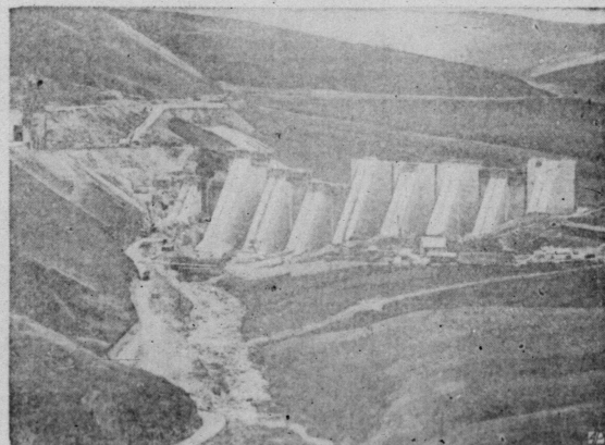
POWER IN THE HILLS — The huge Nantyllyn dam dominates the valley as it rises astride the Rhodri River in Gwynedd, Wales. The dam, part of the Rhodri hydro-electric project, is to play an important role in the economic life of Wales.
