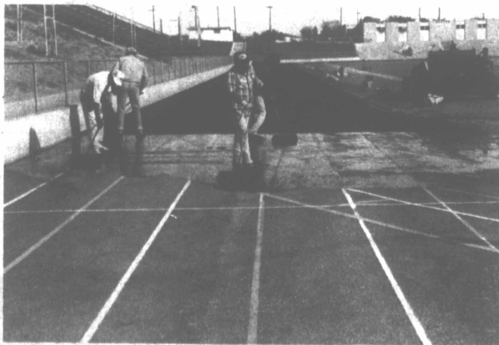
THE TRACK at Wolf Stadium is in the process of receiving a new surface this week as workers from Vibra-Whirl of Panhandle started to work on the project which should be completed Friday or Saturday. Cost to resurface the track, built in 1979, is $44,000.
