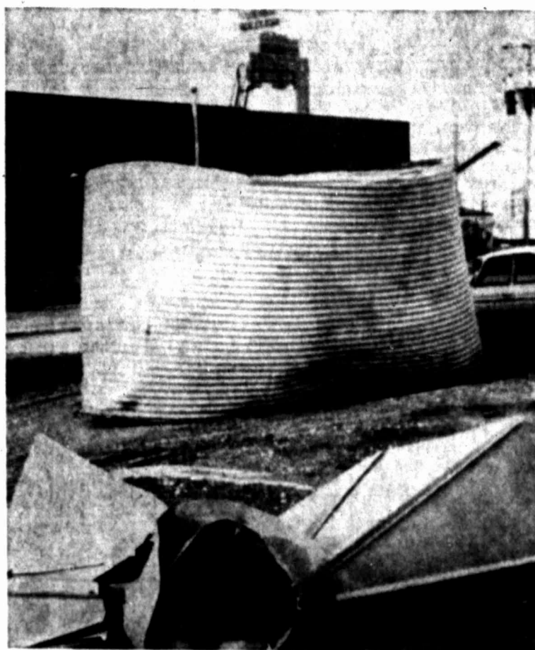
GRAIN STORAGE UNIT CRUMPLED Breckenridge Grain Co., 403 E. 1st
