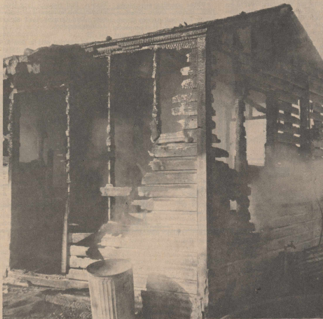
RESULT OF FIRE--Three young children burned to death in this frame home occupied by the James Green family. Cause of the fire which occurred Saturday afternoon was unknown. Rites for the three victims were held here Monday.
