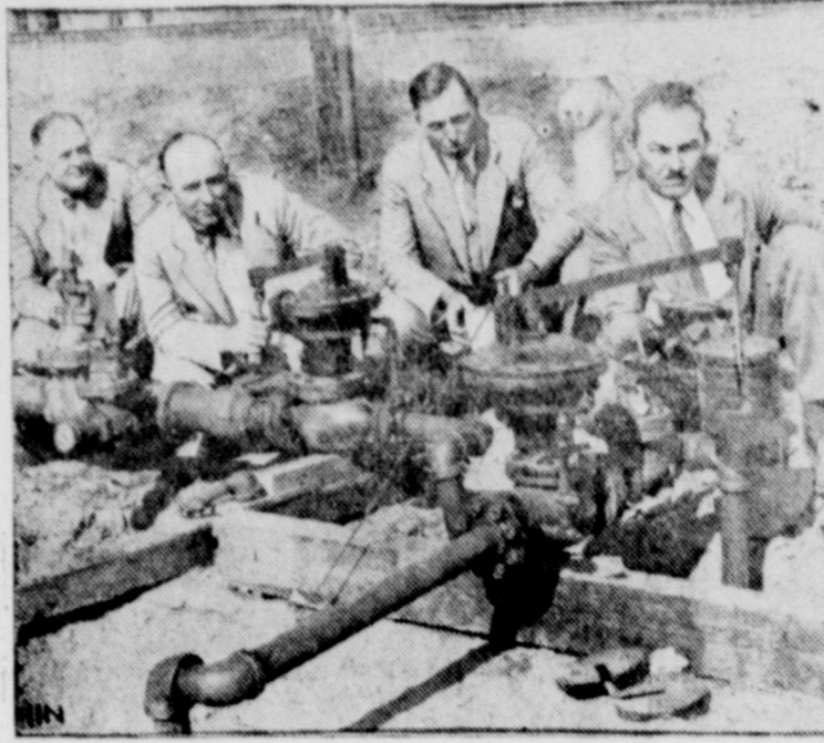
Left to right are John Murry, Lee Horst, H. P. George and Walter Thrall, gas experts, examining the apparatus installed to regulate the flow of gas from the mains as it is blended with pyrofax gas to drive the "Zep's" motors from Mines Field, Los Angeles, to Lakehurst.
