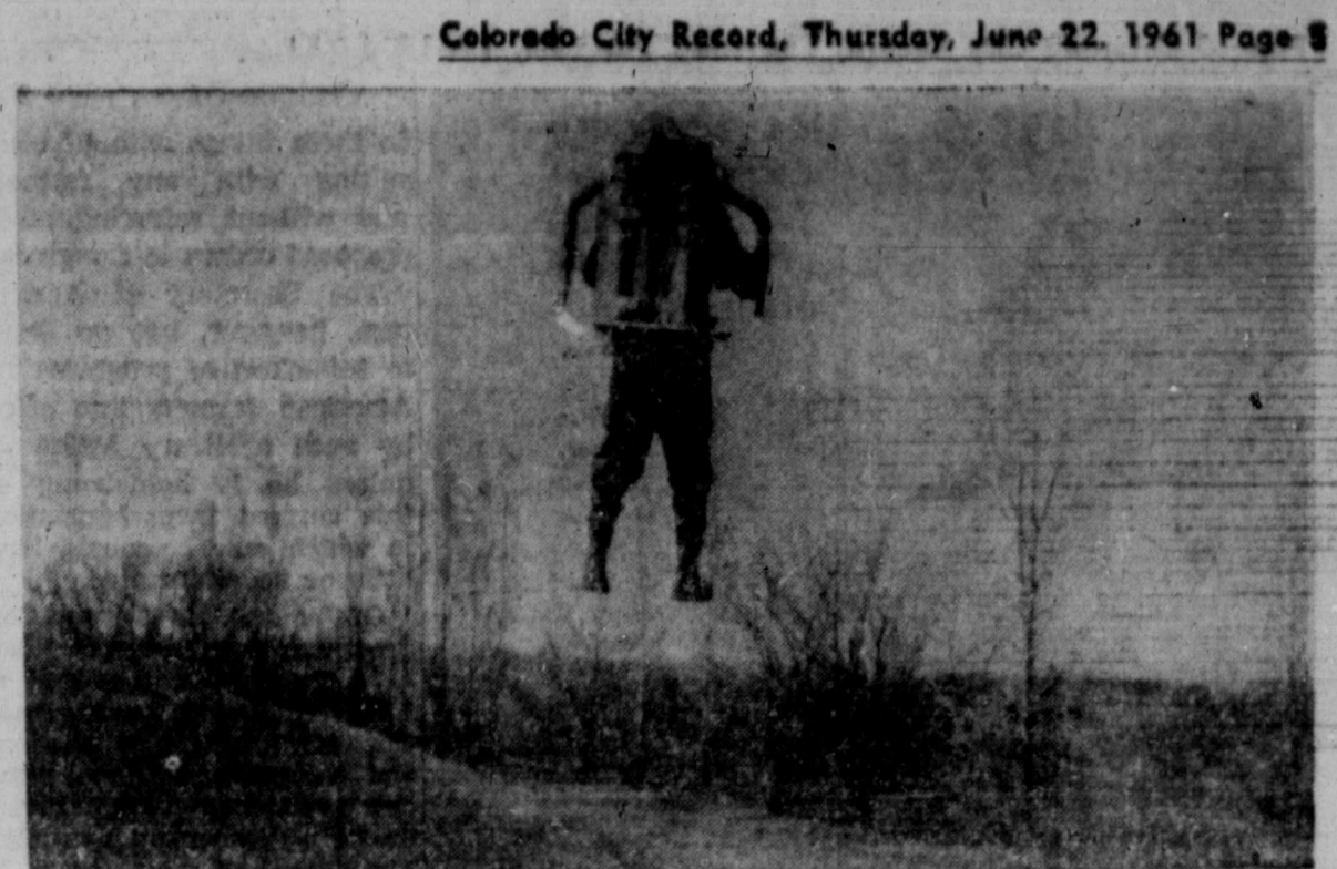
No Visible Means Of Support
