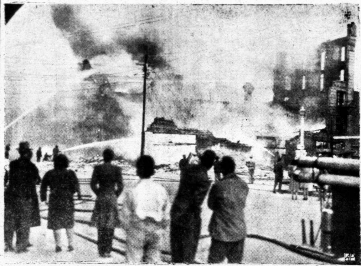
This is the smoking shell of the Texan Hotel at Wichita Falls, Texas, left after an early morning fire swept the seven-story structure; two men lost their lives and ten persons were injured.
