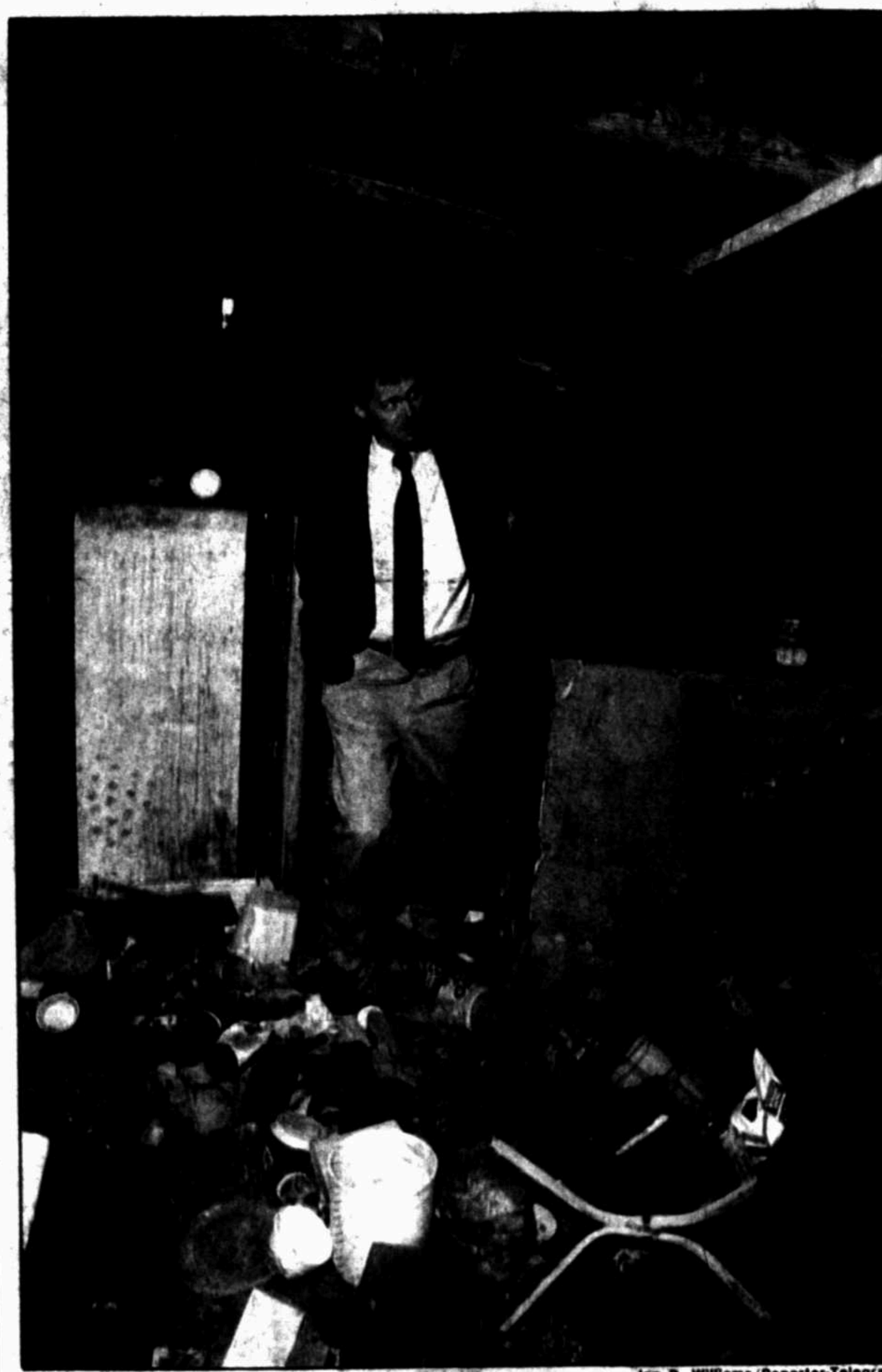
David Wayland, city building official, eyes structural damage and trash in an abandoned house at 500 E. Cuthbert Ave. Thursday.
