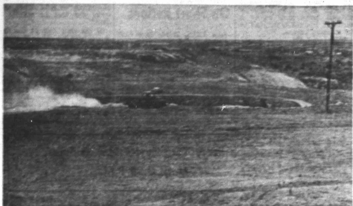
WORK HAS STARTED ... on the first leg of IS 20 bypass
