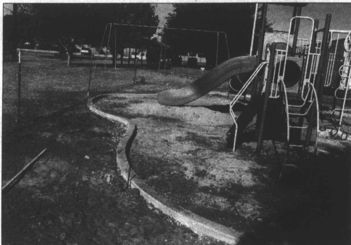
Playground renovation ... Tahoka City Council has approved a master plan to revamp the Tahoka mini park using the half-cent sales tax funds, through the Advancing the Community of Tahoka (ACT) committee. There will be several phases to the changes/restoration until it is complete. Phases 2 and 3 are being done right now. A new curbing and rubber-type ground cover is being put in around playground equipment, and a new shade covering for over the playground will be coming in the next few weeks. Look for more changes throughout the summer. (LCN PHOTO)
