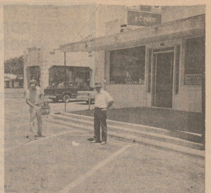
DOWNTOWN PARKING Spaces have been repainted this week by Rolco Traffic Service of Chillicothe. Roland Colmenero, at right, observes as employee Jack Comenoro paints the yellow stripes.
