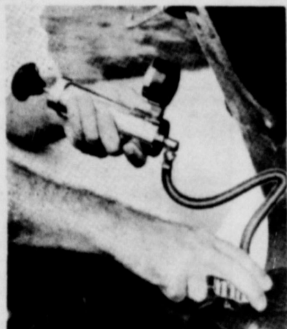
Applying the Tester to the radiator filler neck.
