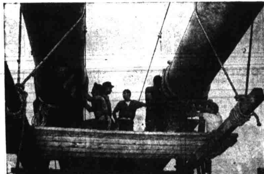
TIGHTENING THE CABLES —Workmen tighten bolts on the cables of George Washington Bridge between New York and New Jersey from a platform that will follow the span.
