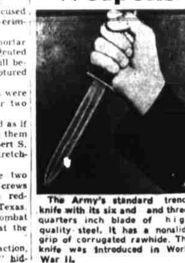
The Army's standard trench knife with its six and three-quarter inch blade of high quality steel. It has a non-slip grip of corrugated rawhide. This knife was introduced in World War I.
