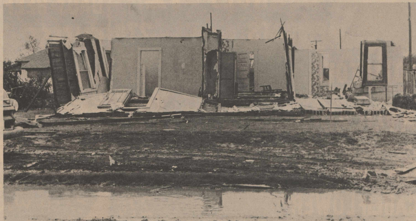
A HOME ACROSS FROM WARD SCHOOL.
