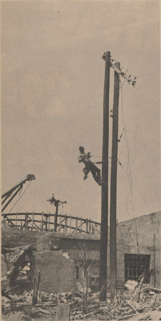
REPAIR BEGINS THE MORNING AFTER.
