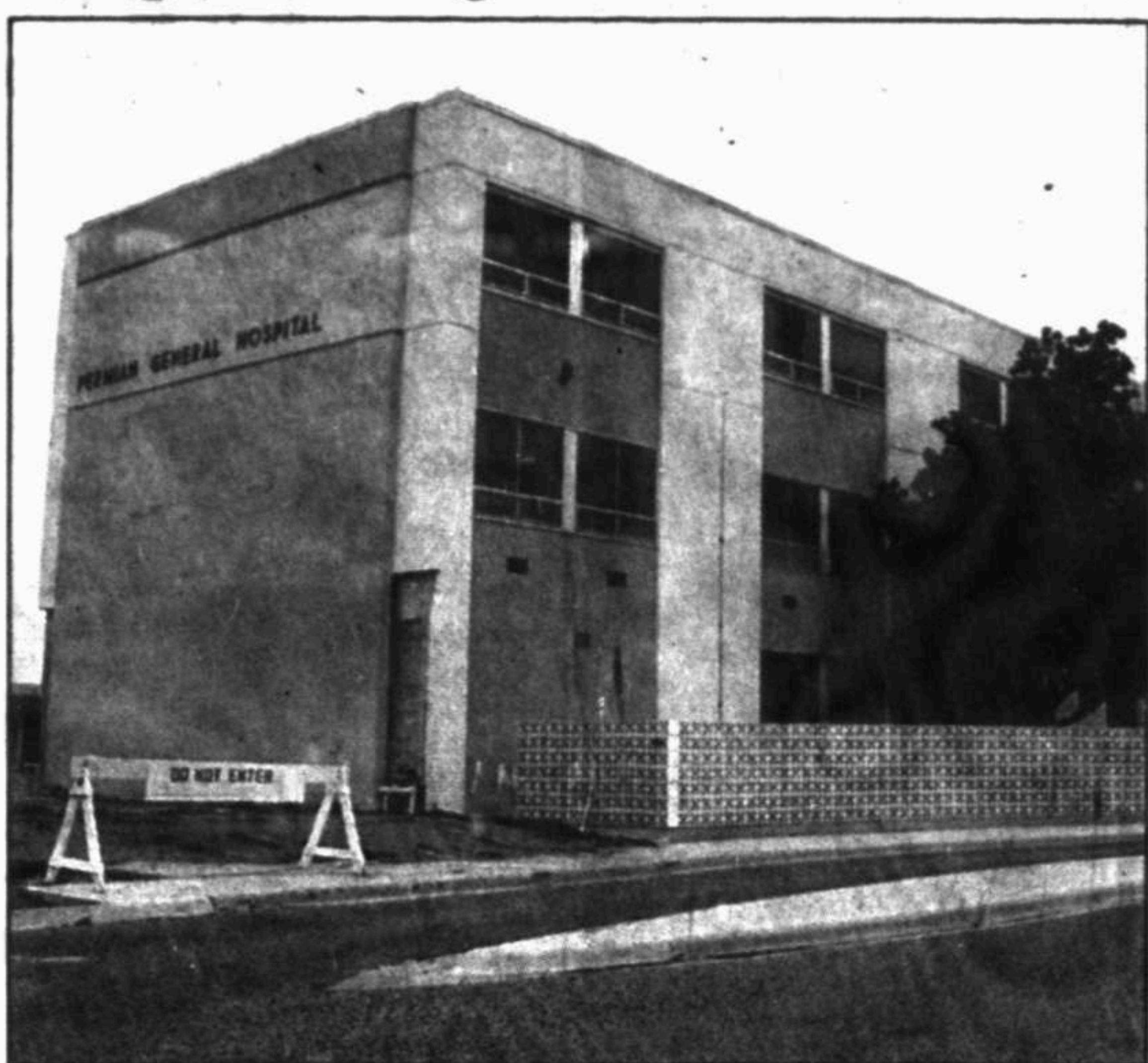
Permian General Hospital, which serves Andrews residents, broke ground last December for a $2.2 million enlargement and remodeling project that will centralize all outpatient services on the ground floor, add an intensive care unit and relocate and double the size of the emergency room. Other improvements will include the enlargement of laboratory, admissions and medical records areas and the relocation of cardiopulmonary.
