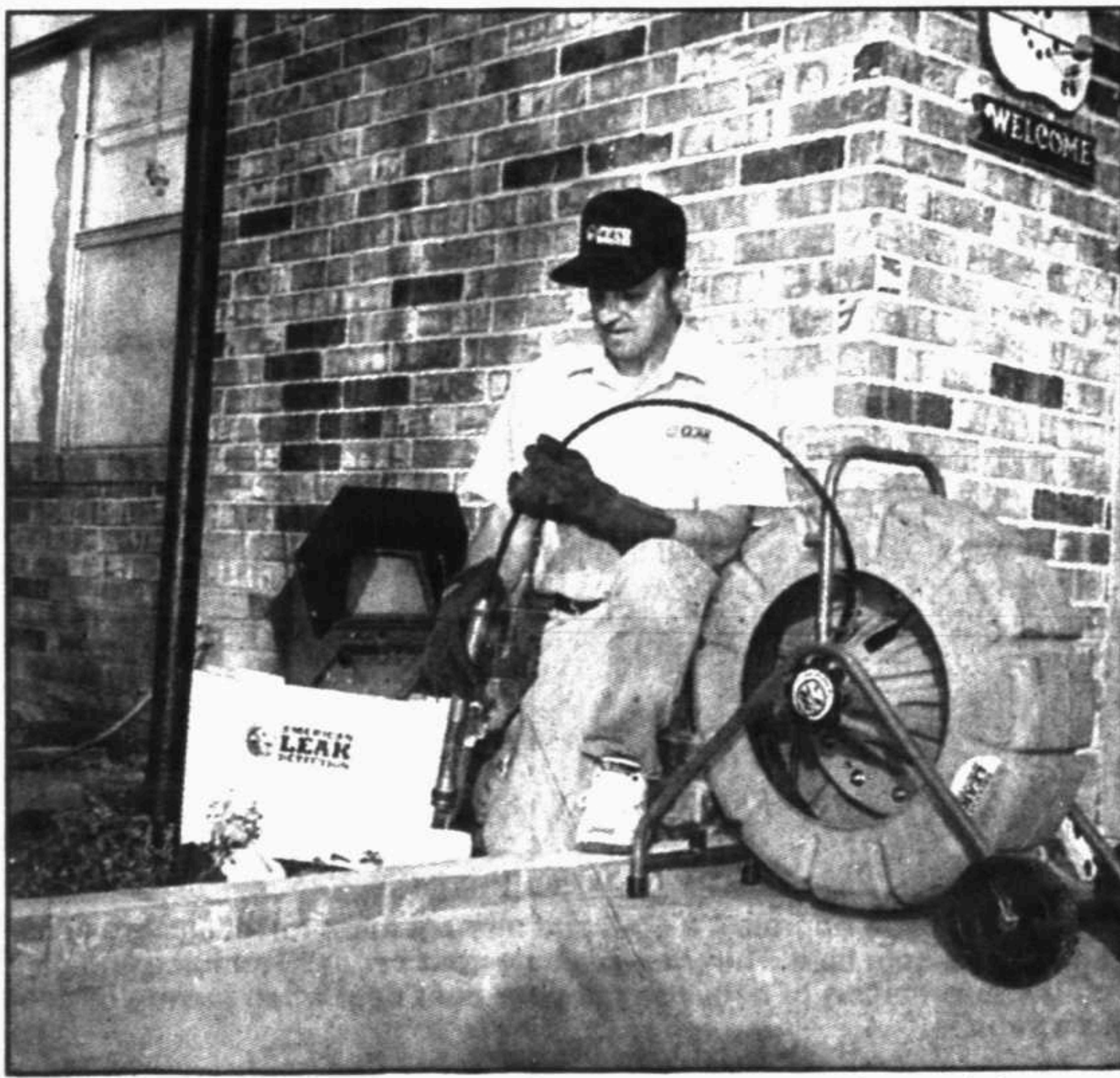
Ricky Lemons of American Leak Detection prepares his special camera to search for sewer problems. Other equipment helps him locate slab leaks, usually within two feet. The phone number is 520-5811.
