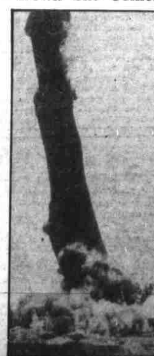
A 200-foot brick stack at an old Lowell, Mass., was wait on the way to oblivion when this photo was snapped. Workmen who pulled out foundation supports to raise it had to make a quick sprint to safety. (Associated Press Photo)
