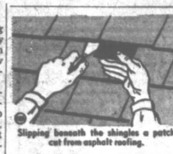
Slipping beneath the shingles a patch cut from asphalt roofing.
