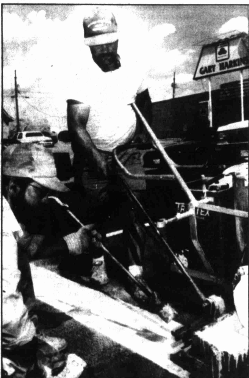
Mark Leist holds a torch to heat the paint as Scott Leist pushes as the duo were painting stop lines Tuesday. The Gregg Street sealcoating project is nearly completed.
