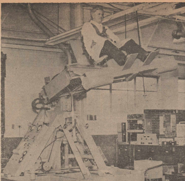
"ROCKING COCKPIT"—Rock n' roll without music is what takes place in this flight simulator moving cockpit mechanism displayed in Belfast, Northern Ireland. Any type flying condition can be tested in the mechanism which swings up and down, from side to side. Does everything but the Twist.
