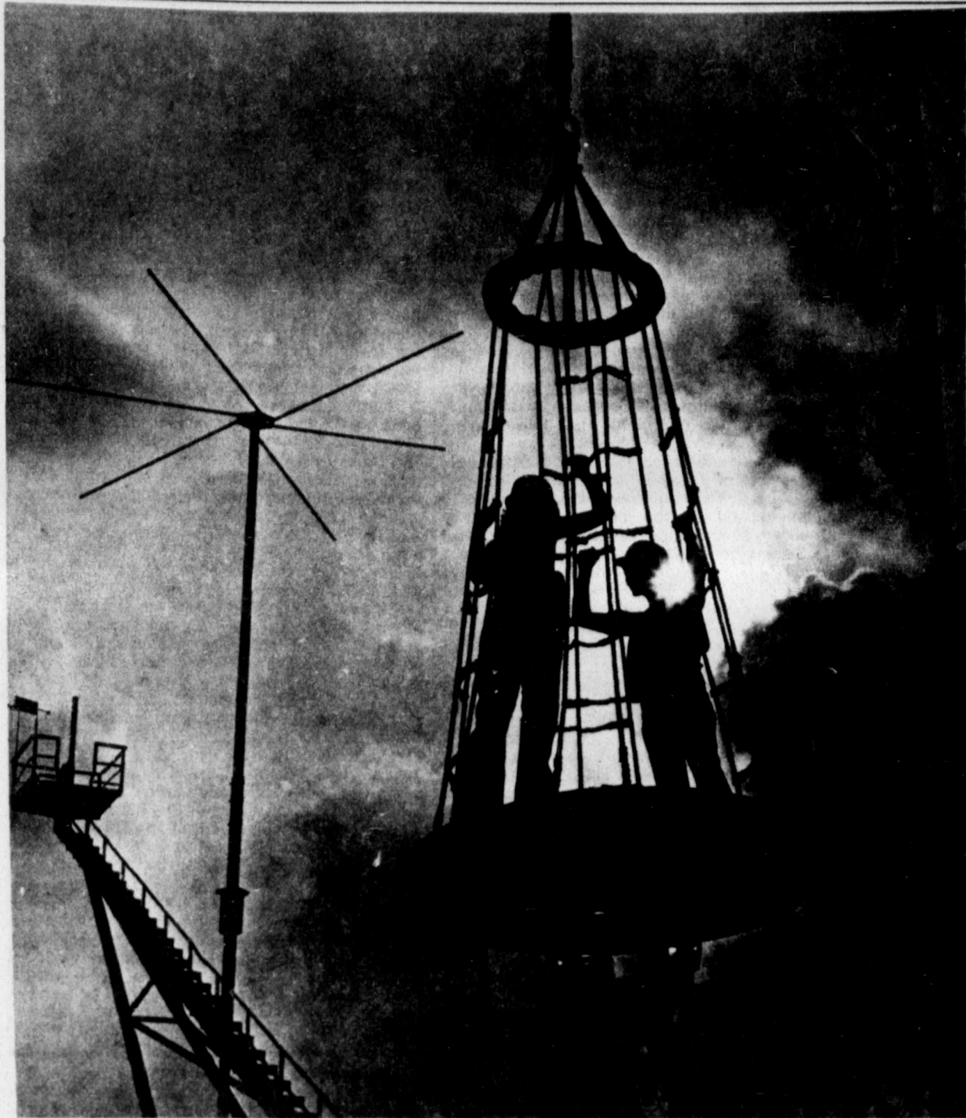
Its nothing like you would find in a fancy office building, but this elevator gets the job done on a Tenneco Oil Co. drilling and production platform in the West Cameron area of the Gulf of Mexico. It is a
