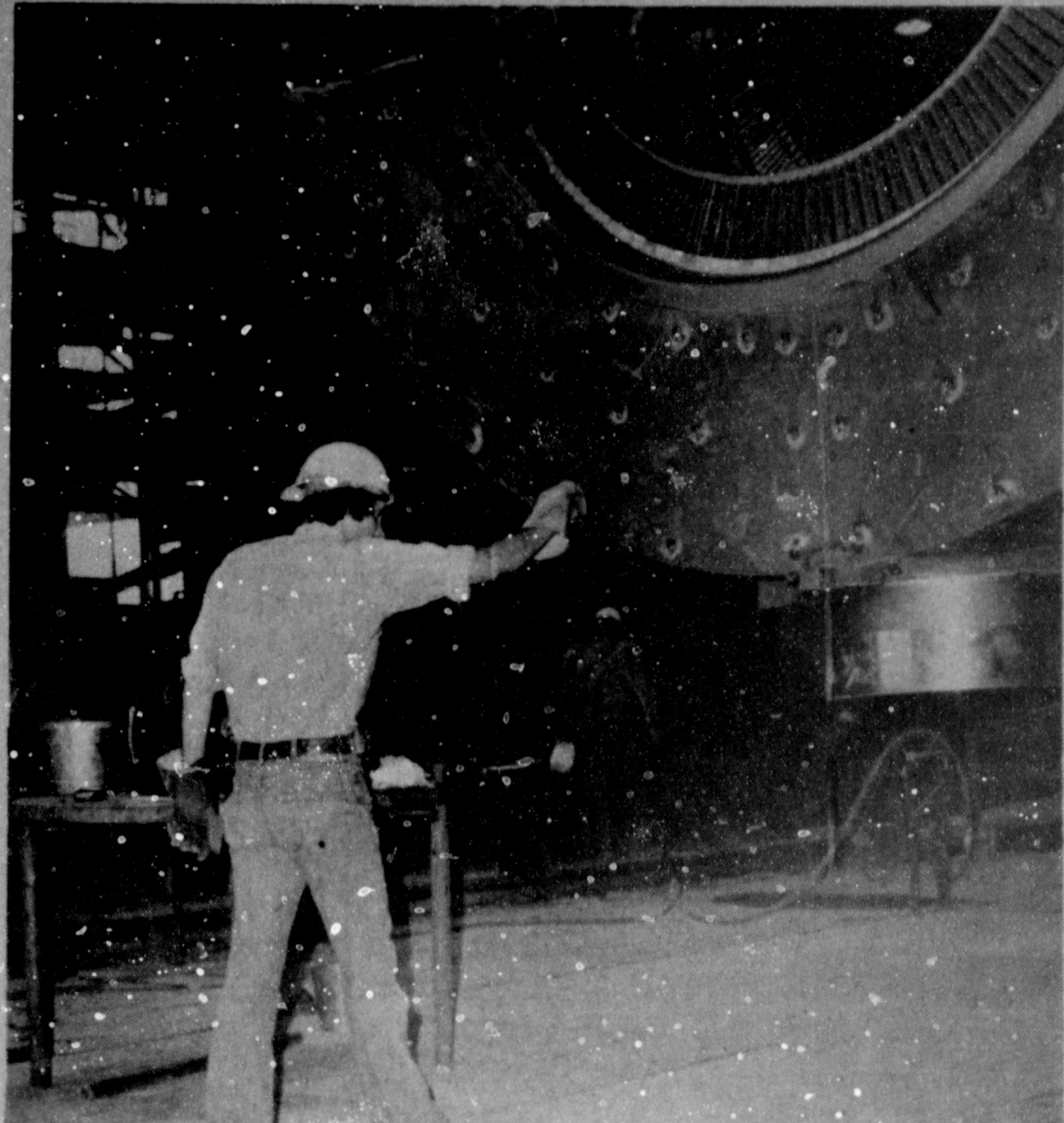
CLOSE SHAVE..... Someone could get a pretty close shave with this turbine blade which is being positioned at the Tolk Station.
