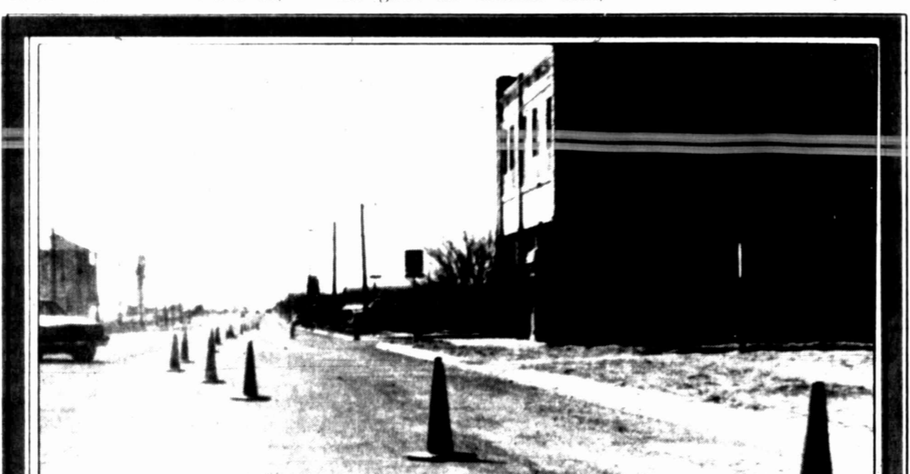
STANTON — A section of U.S. Highway 80 that runs through Stanton will be closed for the next few weeks as workers seal cracks in the road. Officials say it's been at least 10 years since the last paving work was done on the highway.
